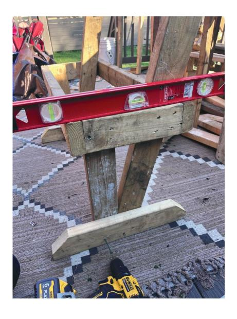
Place 2x8 on box, six inches from the side edge, and the width of a 2x4 over the front edge.
