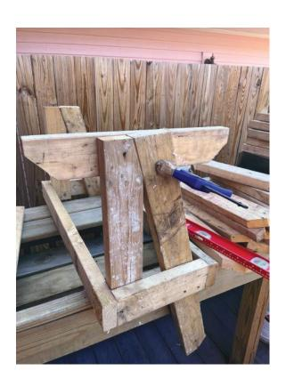
Flip the bench over and set on the ground. Use a level to make it level, then screw in 3 more screws.
