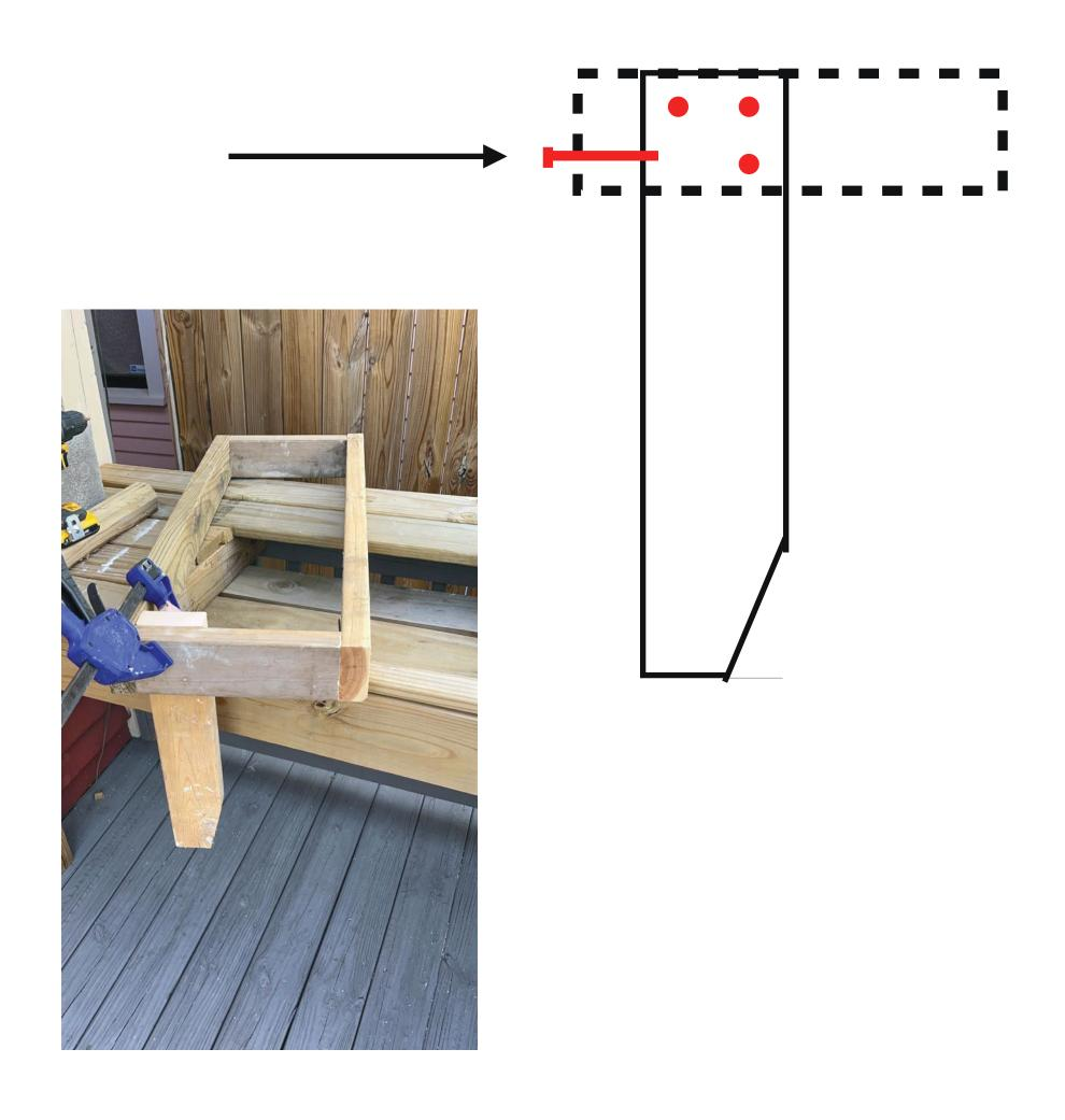
Put the 32 1/4" back leg flush with the bottom of the front leg. Sometimes having the bench upside down on a work bench, using clamps to hold it in place helps.
